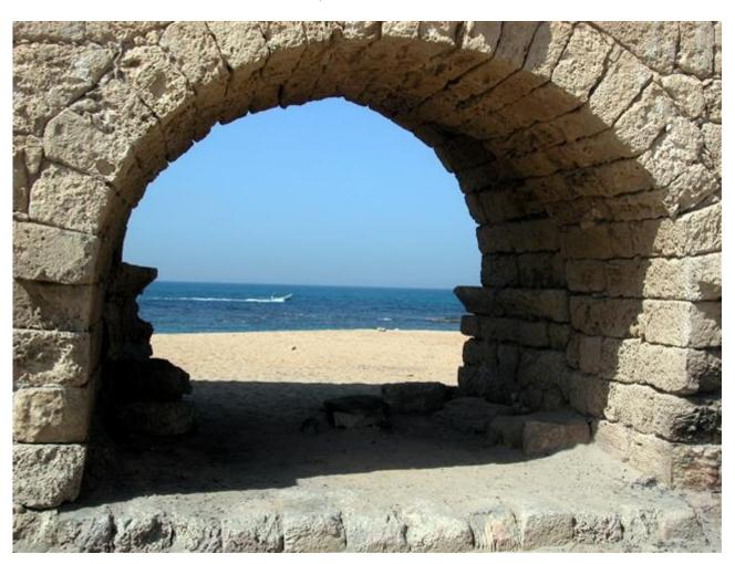
It was constructed with a type of hydraulic cement, invented by the Romans, known as pozzolana. "The Romans found that when they take the volcanic powder found around Mount Vesuvius and mix it with lime and rubble, the substance hardens in water," said Kashtan.
