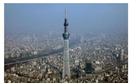
According to the tower's designers, these dampers are capable of absorbing over 50% of the energy emitted by an earthquake. The tower emerged from the 2011 earthquake that hit Japan unscathed, despite the fact that it was under construction by then.
